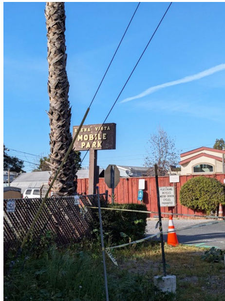
The Housing Authority of Santa Clara County will be replacing Buena Vista's sewer, water, and gas lines, as well as upgrading its electrical grid and repaving. Photo by Myrna Rochester.
