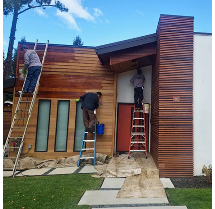
A Cal Preserving crew works on restoration of this wood exterior. Photo courtesy of Cal Preserving.
