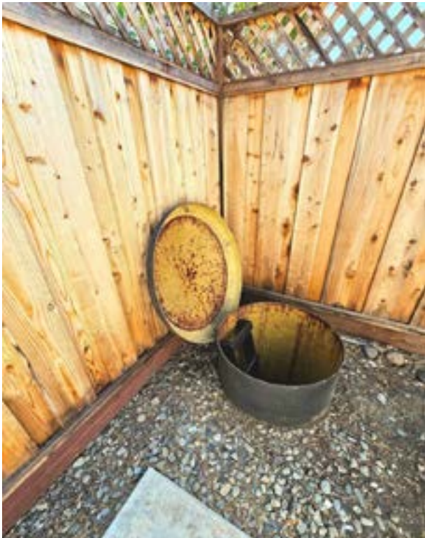
A – Shelter entrance in the side yard between the lot line on the left and the house (out of sight to the right). The underground shelter is about seven feet below the surface of this photo, about 12 feet into the front yard. Photos A, B, and C were taken in July 2025 by Tony Graham.
