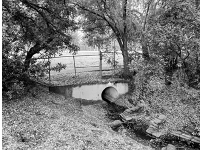
G – Barron Creek culvert outfall at Los Robles Avenue. This is the lower (east) end of the culvert under the Gunn playing fields, at the Barron Park boundary. The photo is taken from the extreme upper (west) dead end of Los Robles Avenue, where a gate permits pedestrians and bicyclists to enter the school property. The pipe looks small in the photo, but it is five feet in diameter. This photo was taken in June 2025, but the scene looked very much the same in 1970 since this channel has been kept clear of vegetation.
