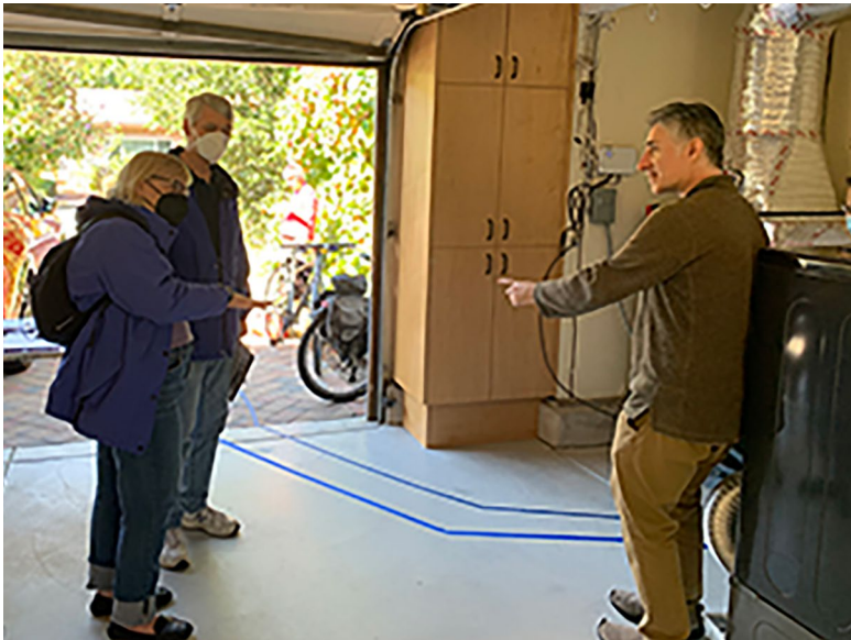
Cedric de La Beaujardiere discusses his heat pump water heater and ground source heat pump with neighbors during the October 14 Peninsula Electric Home Tour. Cedric and Susan Stansbury's home was among four Barron Park homes open to the public during the tour. Photo by Susan Stansbury.
