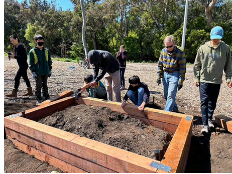
Success on the following beautiful workday as the box is constructed.
