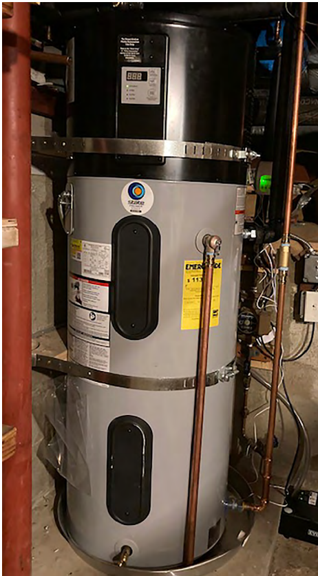
The City of Palo Alto will offer new “heat pump” electric water heaters via a turnkey purchase and installation program starting in early 2023. These new water heaters are over 300% more efficient, smarter, safer, and less expensive to own than gas water heaters. With a mixing valve, they can also “store” excess solar energy in the form of very hot water that can be used when the sun goes down. Photo by Hilary Glenn.
