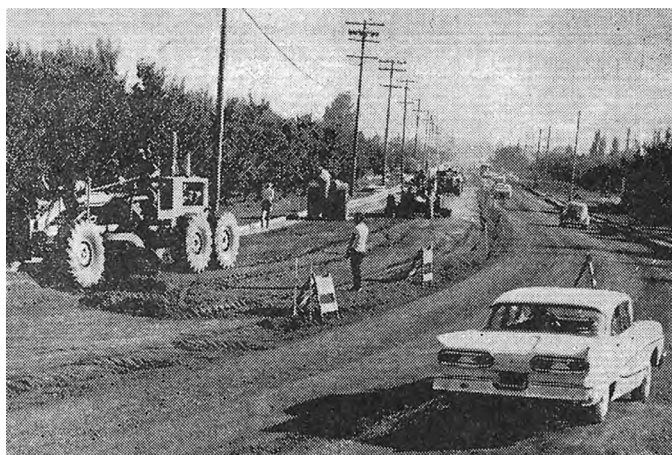
Arastradero Road widening project work, August 23, 1963, looking east (toward El Camino Real) from the curve near the Alta Mesa Cemetery entrance. Photo from Palo Alto Times , from the Palo Alto Historical Association (PAHA) clippings files.
