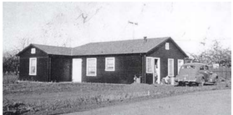
D - 1949 photo of 771 Encina Grande, built in 1949, looking south toward Amaranta Avenue.
